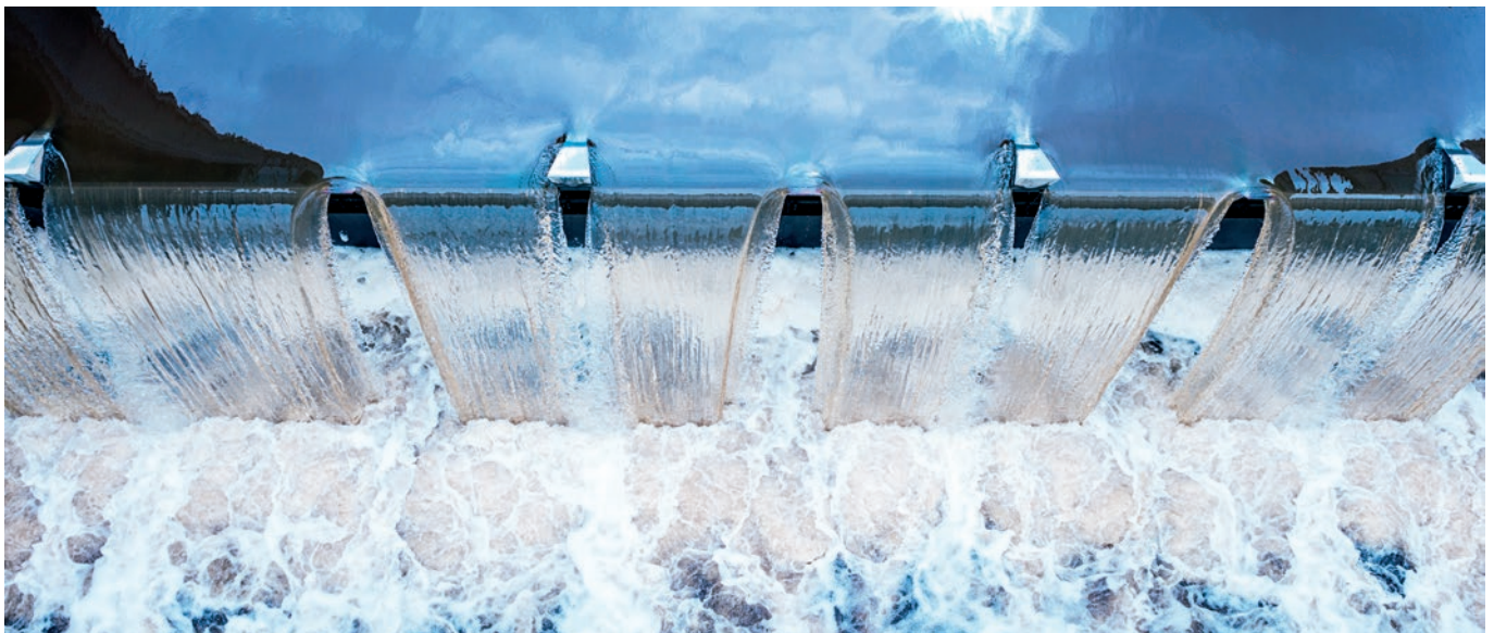
Figure 18. Renewable and flexible hydropower is important for covering the needs of both short- and long-term flexibility. Photo: Statkraft
